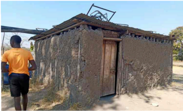
This is the structure that is currently being used as a boys' boarding facility at Kalobolelwa Secondary School
