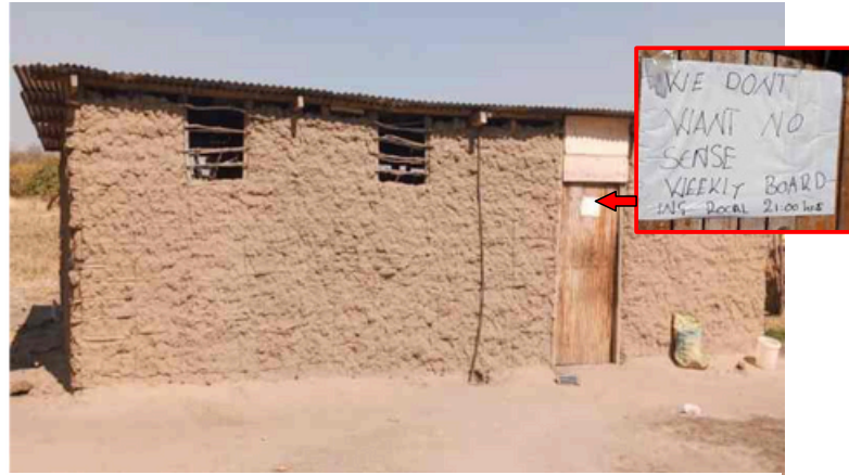
This is the structure that is currently being used as a girls' boarding facility at Kalobolelwa Secondary School
